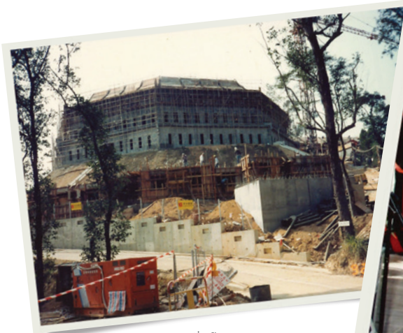
▲ Campus in constructing
